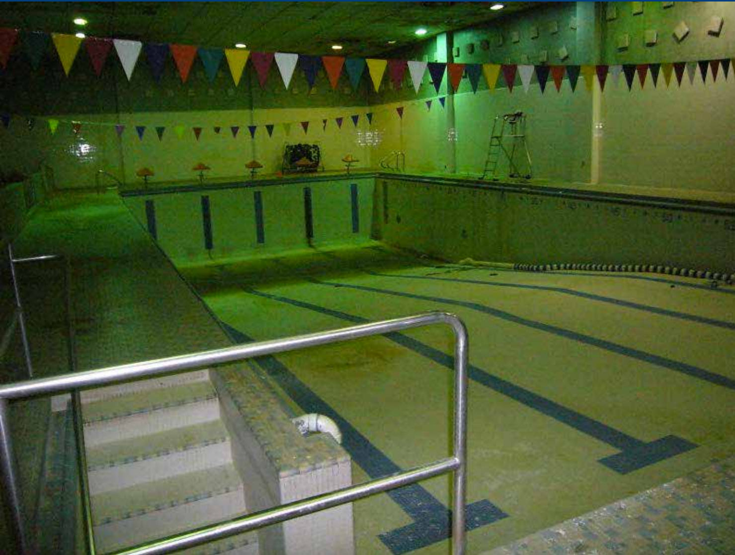
Interior view – Pool
